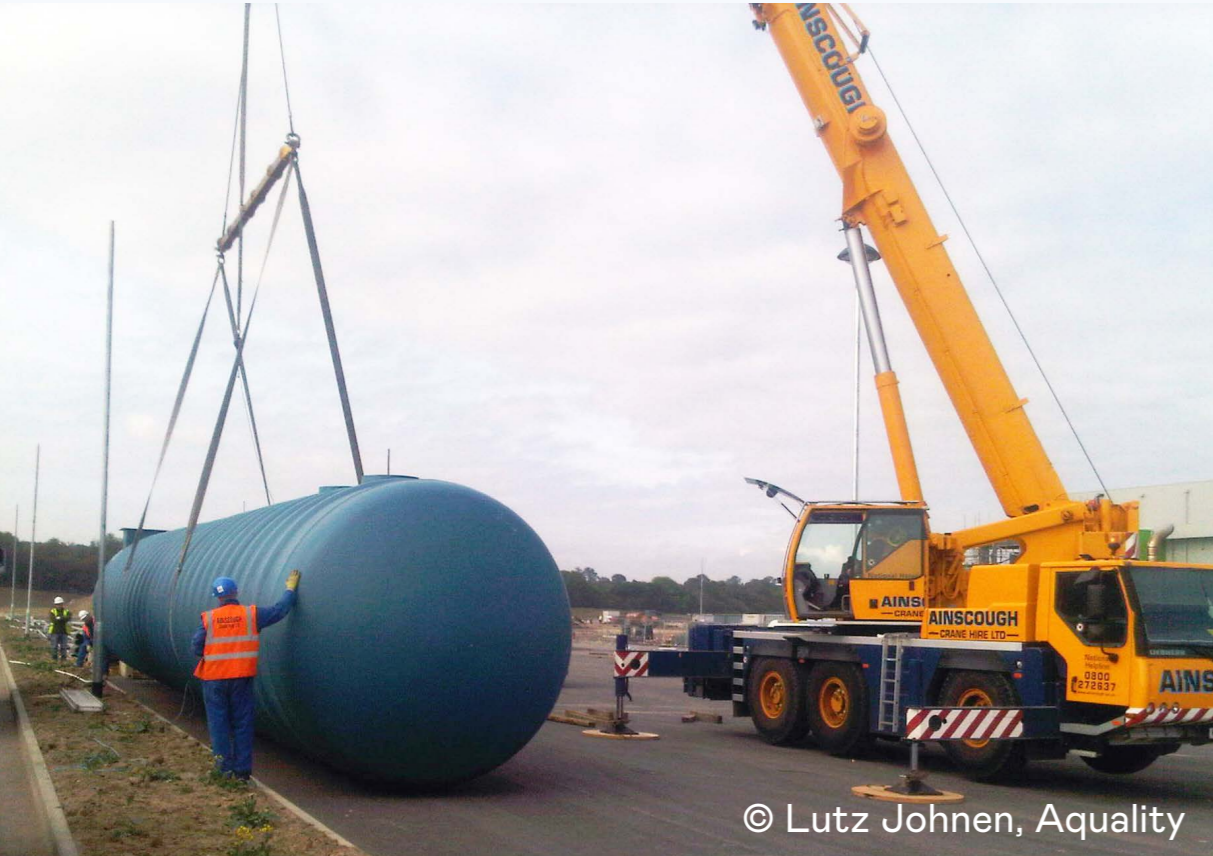
Large scale communal rainwater tank being installed
